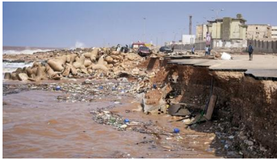
Fig. 7. Collapse of the sewer system after the storm.
